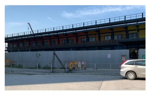
Photo 2 – Erection of site hoardings in unobtrusive colours
