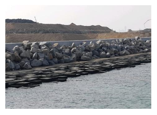
Photo 3 - Natural Rock Material/ Planting for Artificial Seawall
